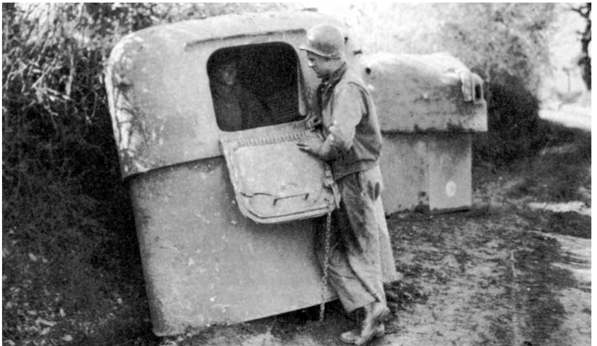
GERMAN PORTABLE PILLBOXES. Some of these were found in the Gustav Line around Cassino and others were later found in the Hitler Line in the Liri Valley. These steel pillboxes, camouflaged and usually connected by communication trenches to well constructed bunkers, were impregnable to all but direct hits from artillery fire. (German mobile steel pillbox, being removed by tank recovery vehicle M31.)
