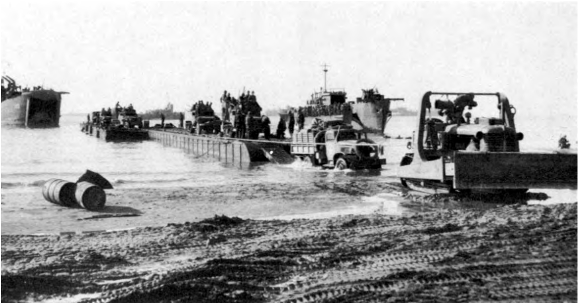
MORNING OF D DAY. Top: men coming ashore from LCI's. Enemy air raids started at 0850 and consisted of three separate attacks by an estimated 18-28 fighter-bombers. One LGI was hit and is shown burning. Bottom: LST backing away from portable ponton causeway after having unloaded. Bulldozer is holding causeway in place. In background is an LGI with a deckload of soldiers waiting to go ashore.
