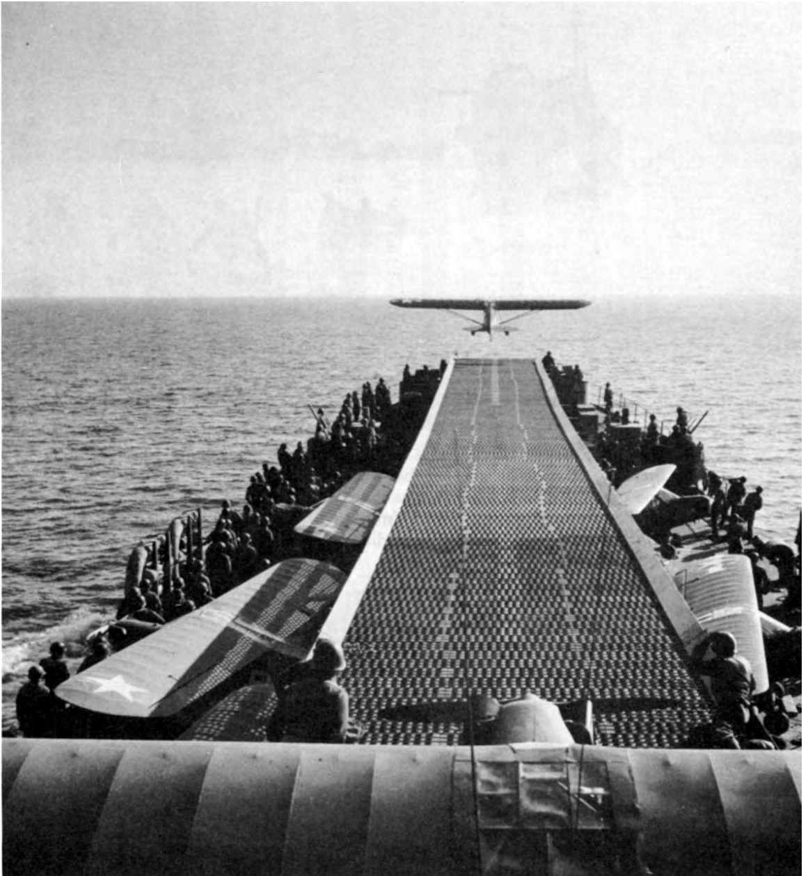
ARTILLERY OBSERVATION PLANE taking off from LST carrier to land at Anzio beachhead shortly after dawn on D Day. The first use of an LST carrier for this purpose was during the invasion of Sicily. Two planes were launched and directed naval fire to the vicinity of Licata, Sicily. Cub planes were to play an important part at Anzio. The area of the beachhead and surroundings is generally flat and featureless and in such terrain observation was at a premium and it was vital to secure or deny that observation.
