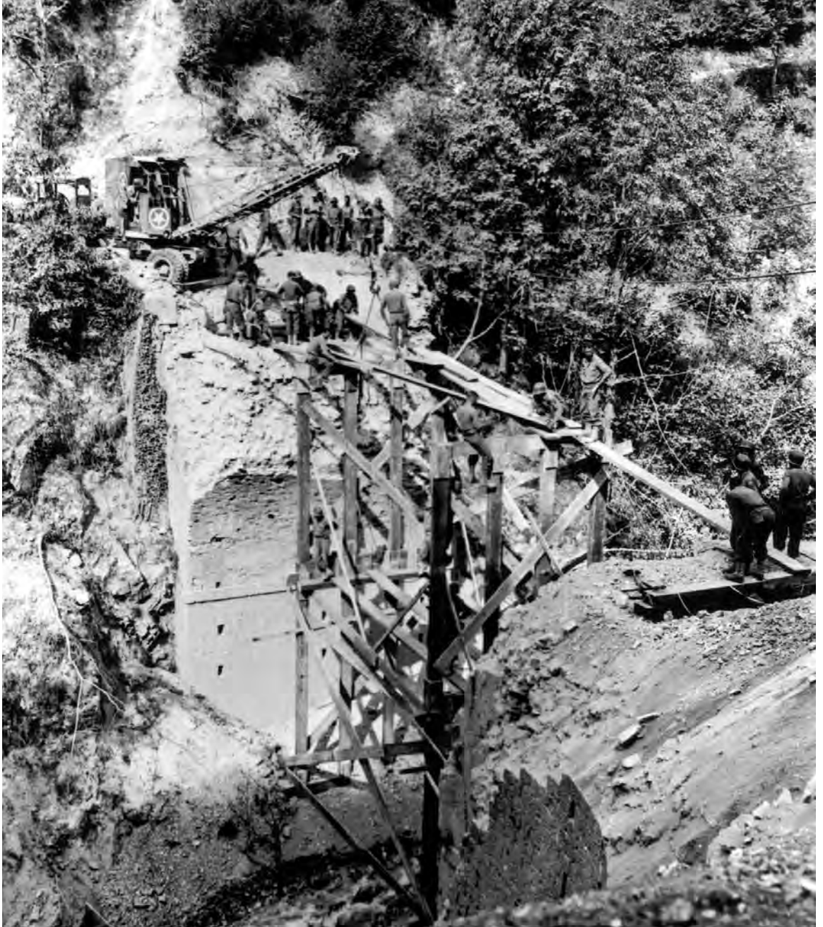
ENGINEERS REPAIRING A BRIDGE NEAR ACERNO. While part of the invading forces advanced westward toward Naples, part proceeded toward Benevento to the north. The enemy retreated slowly toward the river Volturno, the next natural line of defense, leaving rear guards to delay the advance, mine the roads, and blow the bridges.
