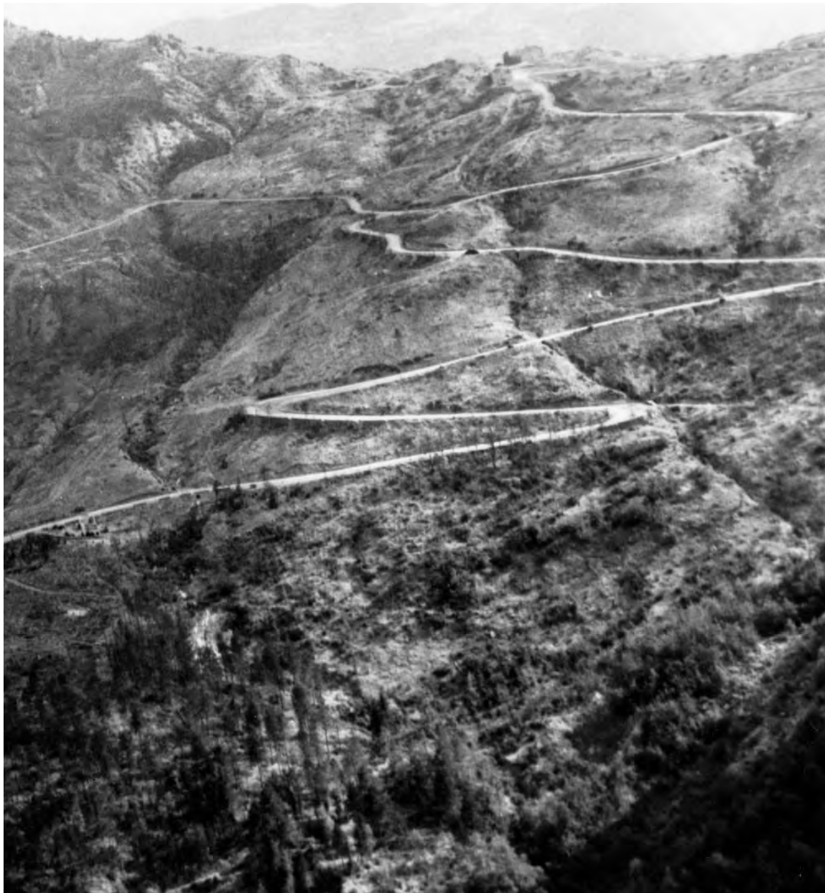
TOP OF IL GIOGO PASS IN THE GOTHIC LINE, looking toward the north. The Fifth Army broke through this pass in the Gothic Line defenses outflanking the heavier prepared fortifications at Futa Pass on Highway 65. The scarcity of roads through the mountains made it possible for the Germans to concentrate their defensive works at a few key points such as the Futa and Il Giogo Passes. Highway 6524 branches off Highway 65 thirteen miles north of Florence, winds through Il Giogo Pass, and ends at Highway 9 in Imola (Po Valley).
