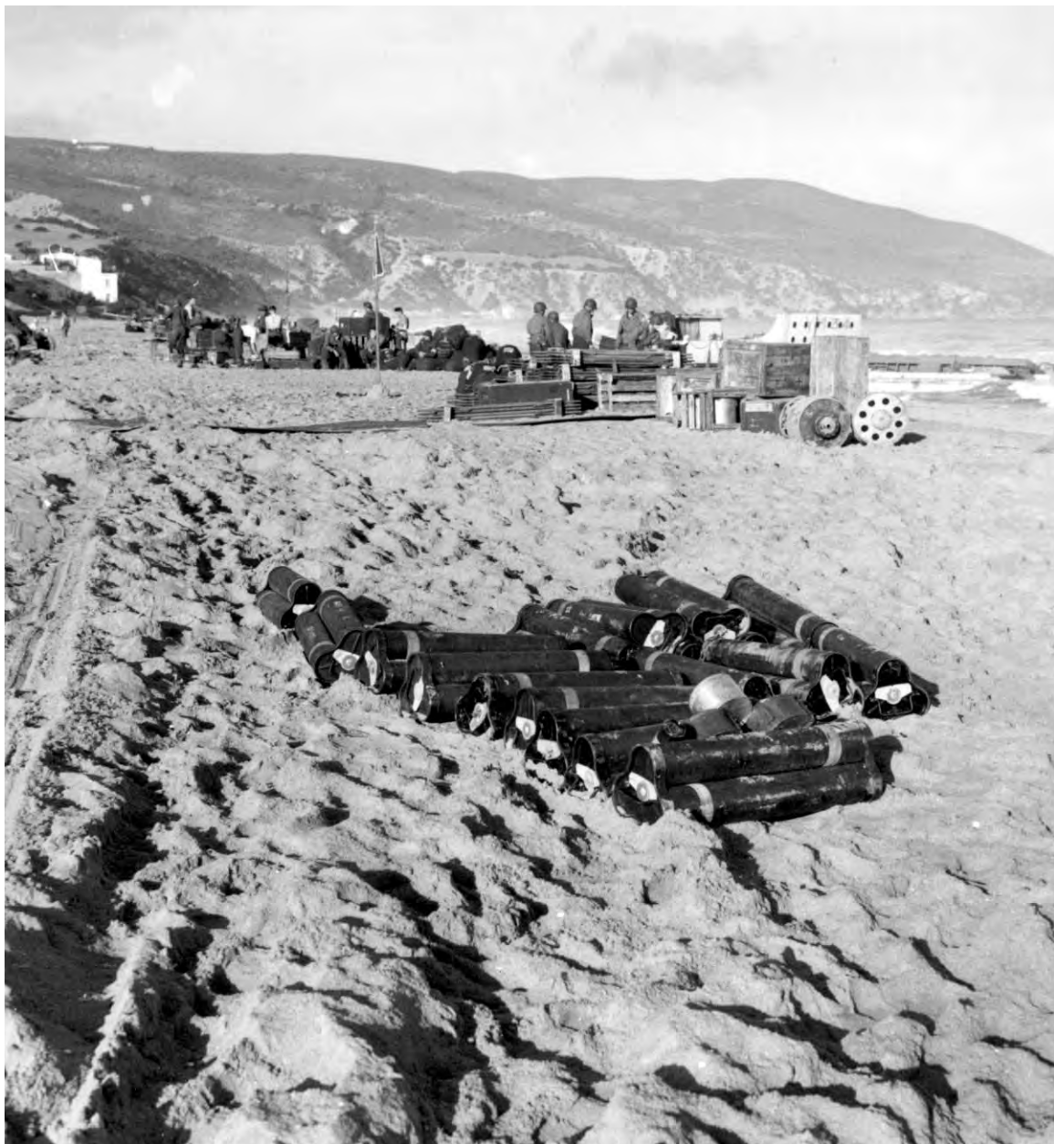
SUPPLIES ON THE BEACH OF LES ANDALOUSES ON D DAY. Most of the Allied supply problems, both on the Atlantic side and in the Mediterranean, were caused by destruction of landing craft. About 95 percent were used during initial landings leaving few reserves for the build-up. The large seaworthy LST's (landing ship, tank), which were to play a decisive role in all subsequent landings, were introduced by the British in the Oran area to carry light American tanks for beach landings.
