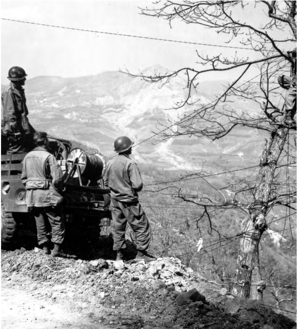
SIGNAL CORPS LINEMEN stringing communication wire in preparation for the coming spring offensive. During the winter stalemate many new lines were strung and hookups were made to the Italian state underground cable system. Circuits linked all units of the Fifth Army and an eight-mile line containing eight open-wire circuits was started in February 1945 from Filigare on Highway 65 near Monghidoro to the village of Lagaro Highway 6620.
