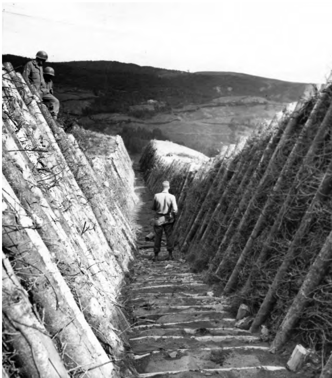
ANTITANK DITCH AT FUTA PASS. This ditch, about three miles long, crossed the road south of the pass. The ditch was covered with a network of infantry positions and bunkers for antitank guns. The area in front of the ditch was mined. Two of the bunkers in this area were topped by Panther tank turrets with long-barreled 75-mm. tank guns.
