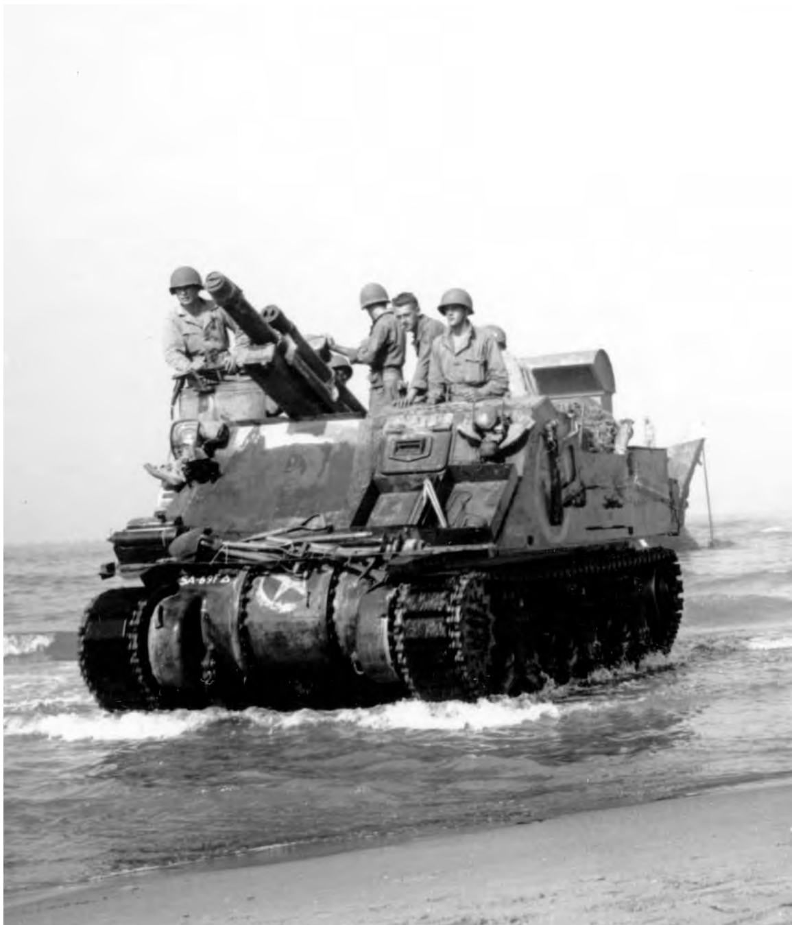
WATERPROOFED PRIEST undergoing test in preparation for the invasion. The invasion training center at Salerno, Italy, established a school of one week's instruction in waterproofing vehicles for the coming assault. The 105-mm. howitzer motor carriage M7 was the principal artillery weapon of the U. S. armored division.
