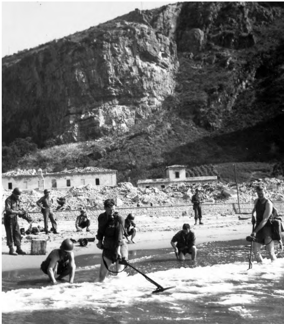
SWEEPING THE TERRACINA BEACH FOR MINES. Terracina is located on Highway 7. During the drive the road became so overcrowded that some supplies had to be shipped by sea. Since the small harbor was cluttered with wreckage of ships, the beach had to be cleared for landing and unloading. (Mine detector SCR 625.)
