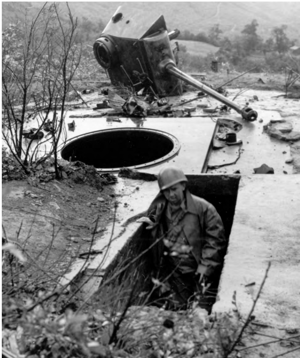
A PANTHER TURRET CASEMATE in the Gothic Line near Futa Pass. The turret could not be penetrated by the guns of any of our tanks, but was vulnerable to artillery fire.
