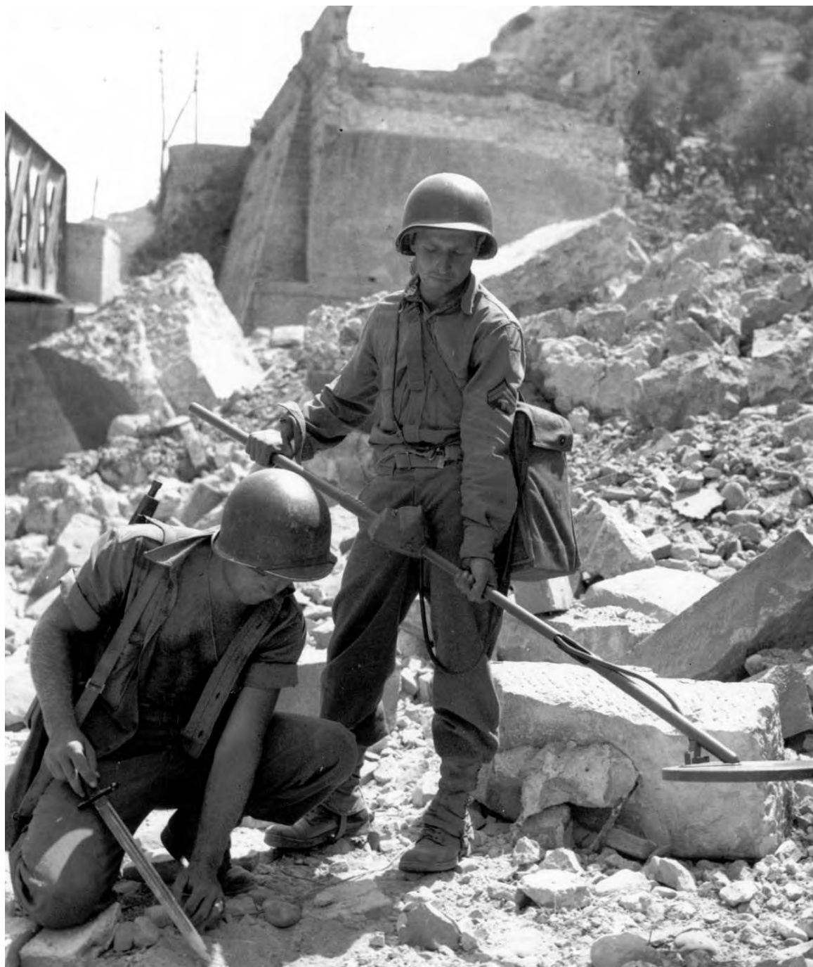
PROBING FOR MINES AT A BRIDGE-CROSSING SITE. The mine detector reacts to metal; whether the metal was a mine or a shell fragment had to be determined by probing and digging, usually with a bayonet. (Mine detector SCR 625.)
