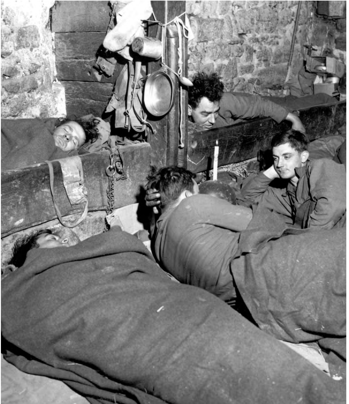
MEN RESTING IN THEIR QUARTERS in an old barn after a day in foxholes at the front. During cold weather, winterization of living quarters was carried out on a large scale, although men in the extreme forward positions usually had to improvise with a raincoat and a blanket in a foxhole.
