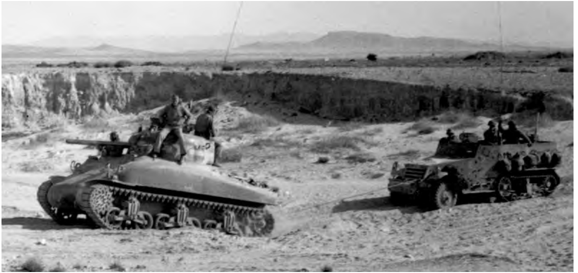
GENERAL SHERMAN TANK TOWING DISABLED HALF-TRACK at Sidi bou Zid (top). This tank gradually replaced the M3 (General Grant) in Tunisia. Its principal weapon was the 75-mm. cannon. Its turret could traverse an arc of 360 degrees in contrast to the sponson-mounted gun on the General Grant with a traverse of about 30 degrees. Reconnaissance party at Kasserine Pass on the Kasserine-Thala road (bottom). The enemy came up this road on his attack through the pass and stopped just before reaching Thala after indications of increasing Allied strength. (Medium tank M4.)
