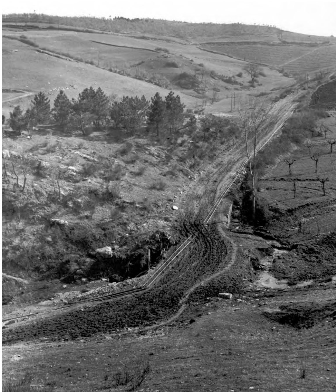
DOUBLE PIPELINE which carried gasoline from the port of Leghorn to the army front in the Apennines. "Pipeline walking" to inspect for leakage was done by jeep whenever possible. Because of hilly terrain several booster pumping stations were necessary. (4-inch double pipeline.)
