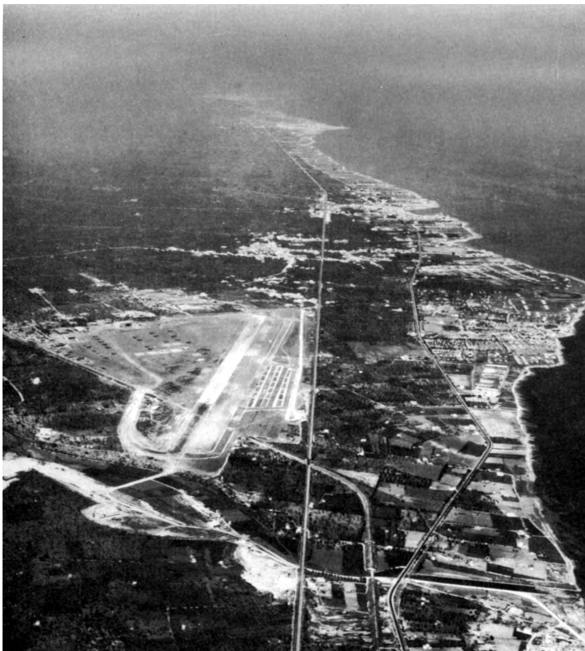
BARI AIRPORT, on the Adriatic just north of the heel of Italy, was captured by the British on 22–23 September 1943. The enemy had used this airport as a transport base and for staging fighters on the way to Africa. The near-by town of Ban became headquarters for the heavy Allied bombardment units based at several airfields on the Foggia plain. Both the town of Ban and the Bari airport were subject to attack by enemy aircraft.
