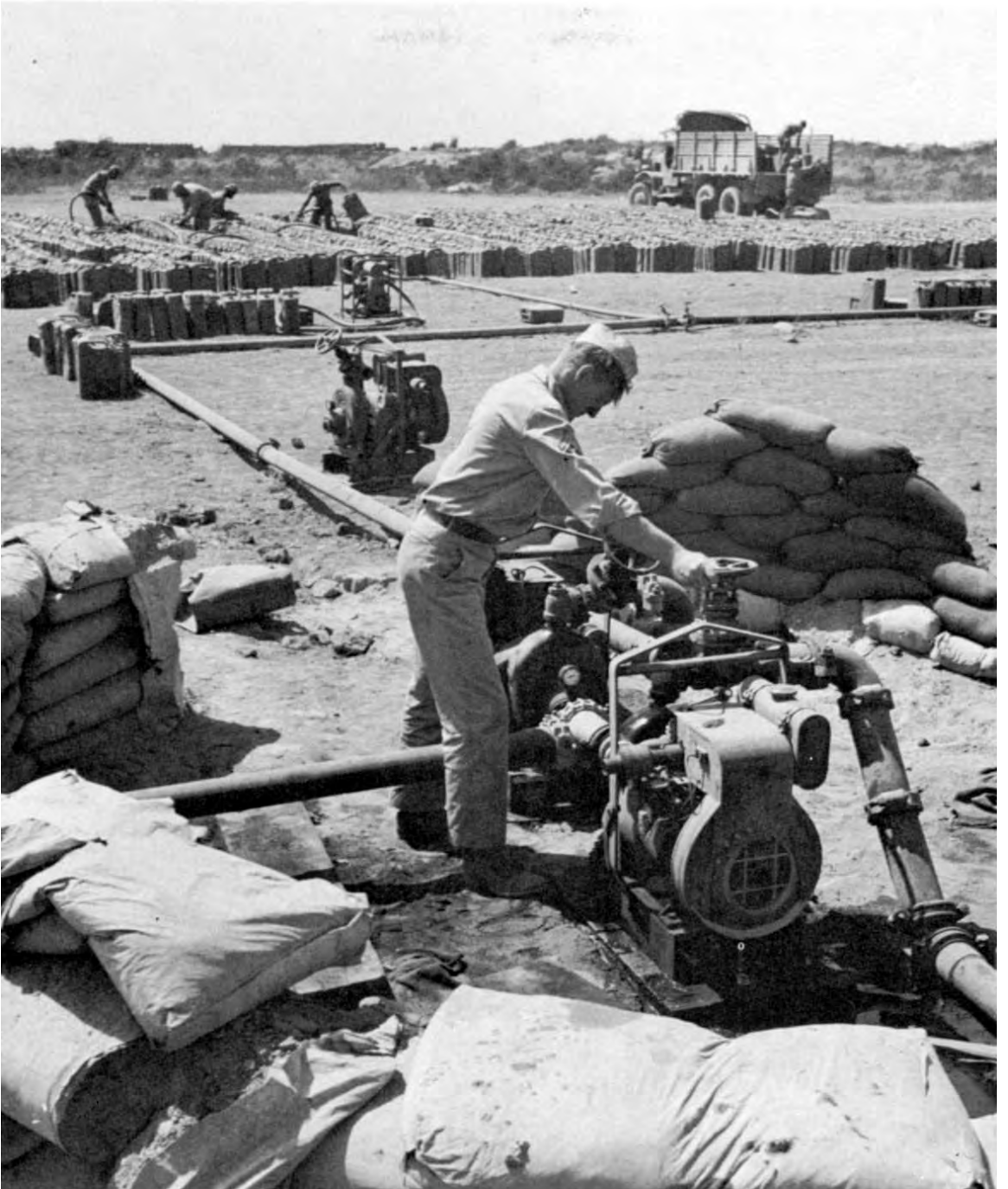
GASOLINE DISTRIBUTION POINT. Oil tankers brought gasoline into major ports. From there it was transported to storage tanks at distribution points by pipeline, trucks, or tankers where it was transferred to five-gallon cans for pickup.
