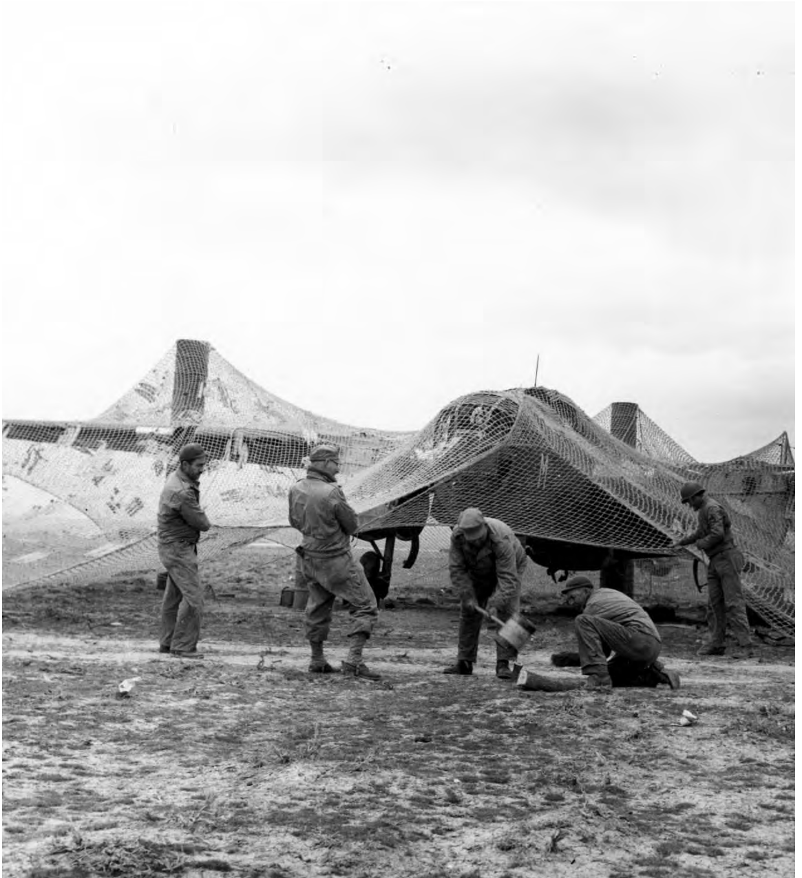
CAMOUFLAGING MEDIUM BOMBER at Youks-les-Bains airfield. Camouflaging for hiding purposes in olive groves or on rough terrain was relatively successful; however, camouflaging an aircraft on a flat, featureless landing field for hiding purposes was not practical. Camouflaging was often practiced to the extent of deceiving the enemy about the type or serviceability of planes. Note that the bomber above is minus both of its engines. (Martin B-26 Marauder.)
