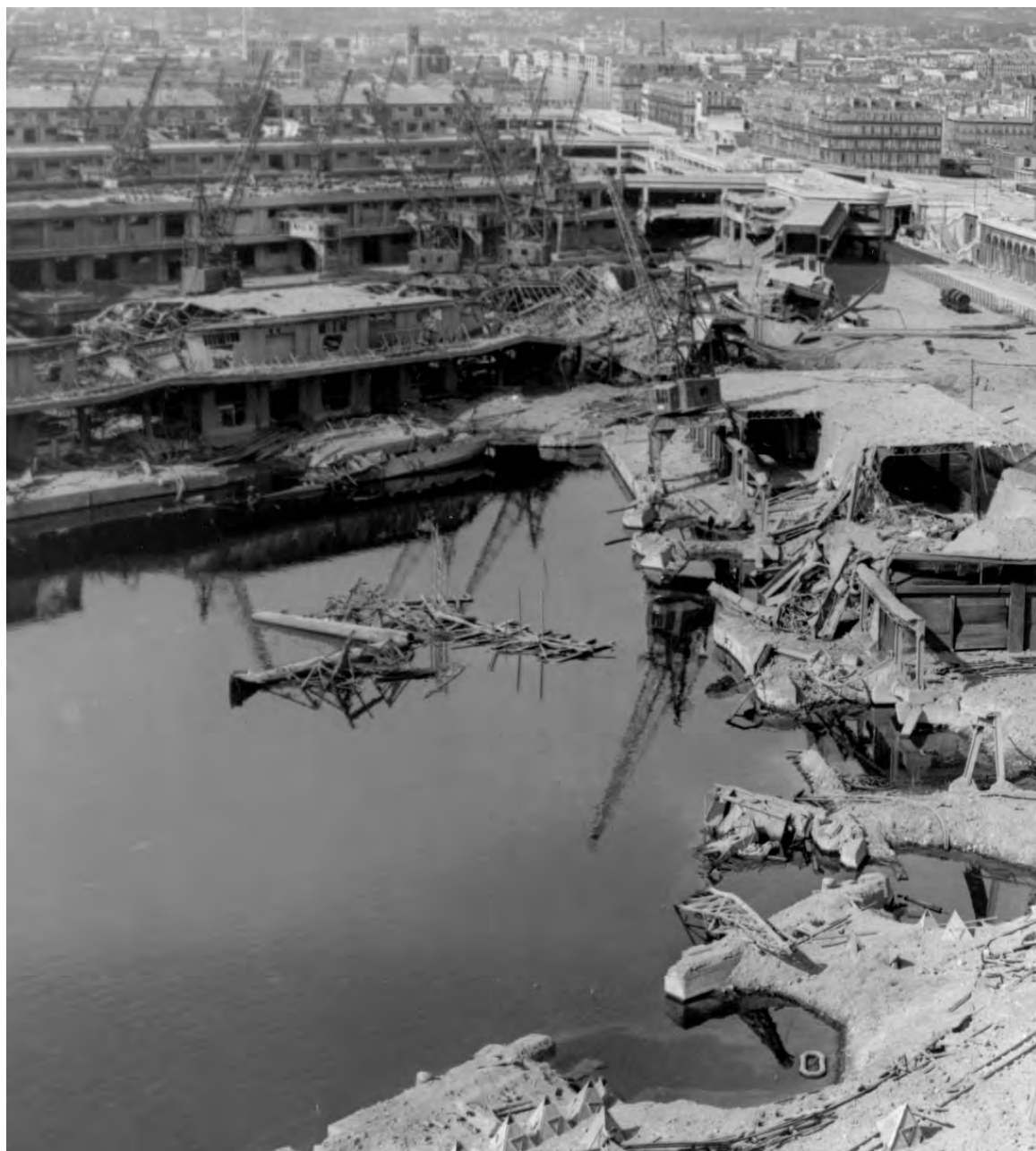
DAMAGED DOCKS AT MARSEILLE, the second largest city in France, the most important port on the Mediterranean, and one of the three cities in southern France with facilities for handling 10,000-ton Liberty ships. (The others are Toulon and Nice.) Marseille capitulated to the French army on 28 August 1944, particular emphasis being placed on preserving port installations which the Germans had hoped to render useless by large-scale demolitions.
