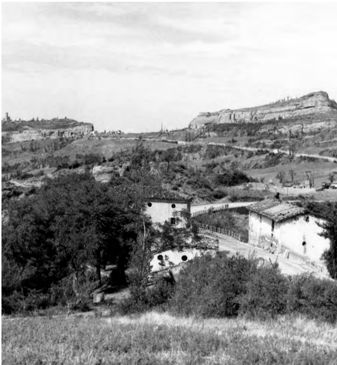
APPROACH TO LIVERGNANO ON HIGHWAY 65, looking from the south along the highway. The village is the small cluster of ruined houses below cliff on left. The Germans occupied the houses as well as the tops and sides of the two hills. The latter were honeycombed with caves which the enemy had enlarged and strengthened. The fighting lasted from 9 to 14 October. On the 14th the enemy was still in possession of most of the village and the two hills but retreated because he had been outflanked from the west.
