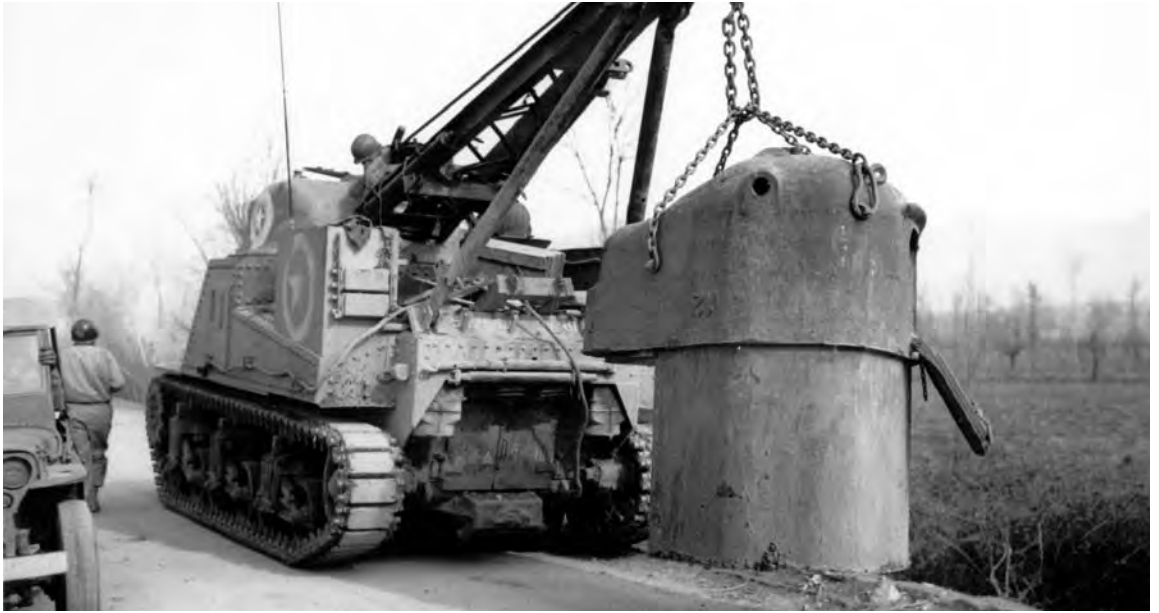
GERMAN PORTABLE PILLBOXES. Some of these were found in the Gustav Line around Cassino and others were later found in the Hitler Line in the Liri Valley. These steel pillboxes, camouflaged and usually connected by communication trenches to well constructed bunkers, were impregnable to all but direct hits from artillery fire. (German mobile steel pillbox, being removed by tank recovery vehicle M31.)
