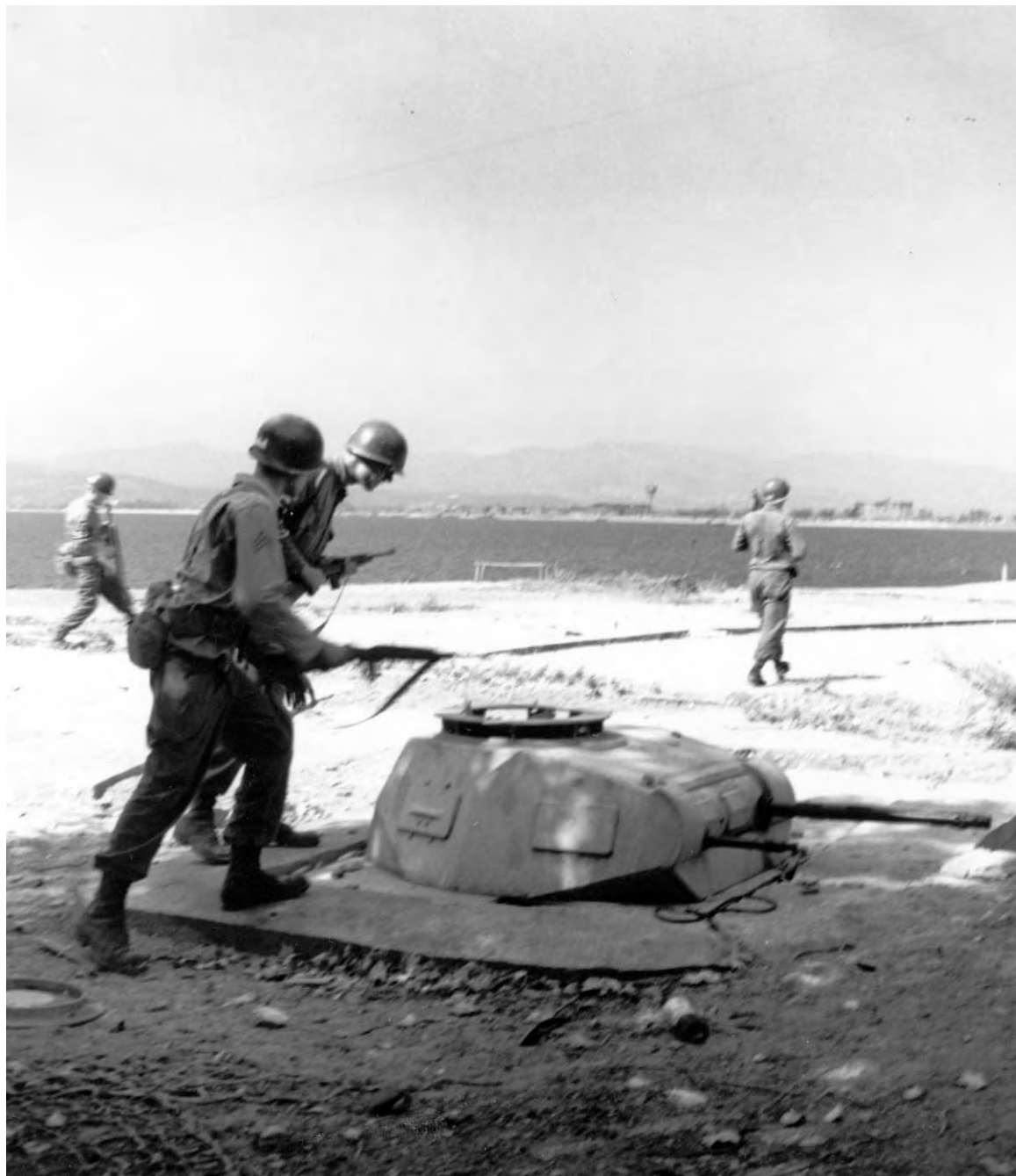
ENEMY PILLBOX. On the morning of 16 August 1944 troops moved through Saint-Raphaël clearing most of the resistance. There was considerable improvisation on the part of the enemy, such as the mounting of tank turrets on concrete to form pillboxes. ( Schmeiser machine gun and 20-mm. cannon mounted in pillbox.)
