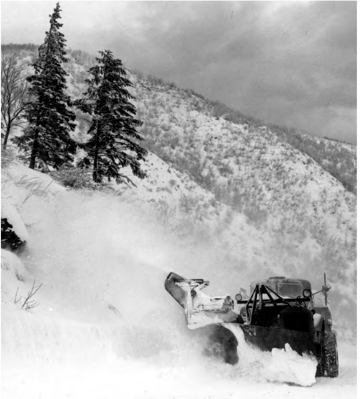
TRUCK WITH ROTARY SNOWPLOW clearing Highway 64 near Collina. The first snow fell in the mountains on 11 November. Snow, rain, sleet, and ice-coated curves on the roads leading to the front made the supply situation a difficult one. The constant work by snowplows and the hand labor of thousands of soldiers and Italian civilians kept the main roads open throughout the winter.
